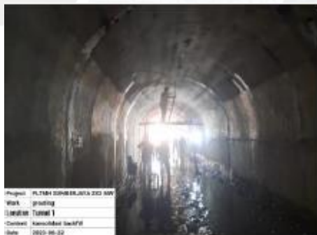
Tunnel Grouting Backfilling
