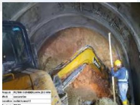
Tunnel Excavation Outlet, Pouring concrete cyclops,
