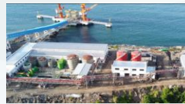
GLP Coal Jetty
